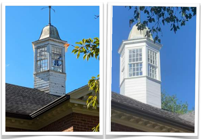
Recent work at the Library includes restoring Weaver's cupola. Left, before; right, the renewed feature.
